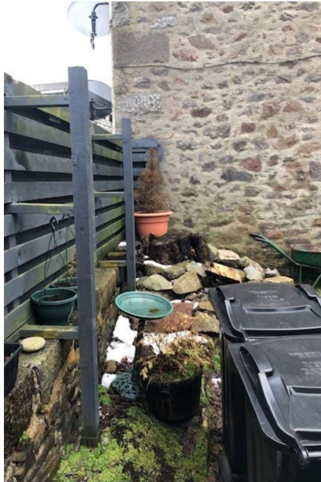
Existing fence/wall (facing south)
