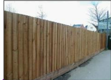
1.8M HIGH CLOSE-BOARDED TIMBER FENCE
