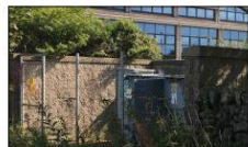
EXISTING SUB-STATION GRANITE WALL RETAINED AND REPAIRED AS NECESSARY
