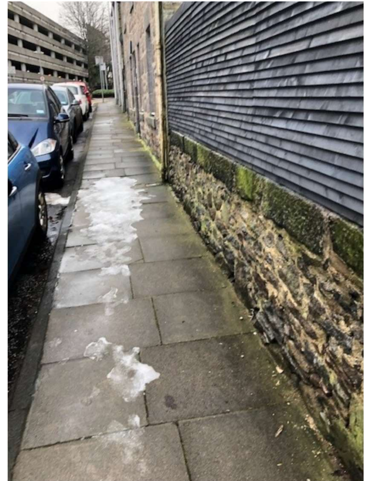
Boundary wall & fence (facing south)
