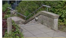
EXISTING FACING BLOCK/GRANITE WALL RETAINED AND REPAIRED AS NECESSARY
